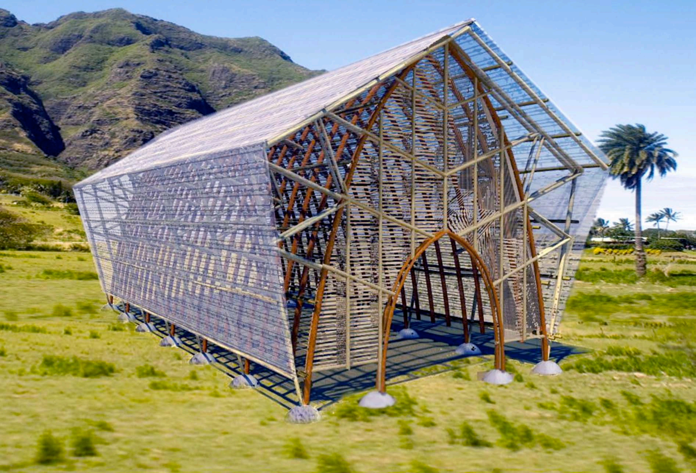
The Main Hall is another structure flanking the Main Plaza. It is a blend of futuristic high -tech materials (Solar Membrane) and Terra Nova harvested bamboo. The bamboo was assembled into a truss system, repeated to create space, and covered by solar membrane to provide full power and protection from the elements. It is Terra Nova's social gathering hall.
